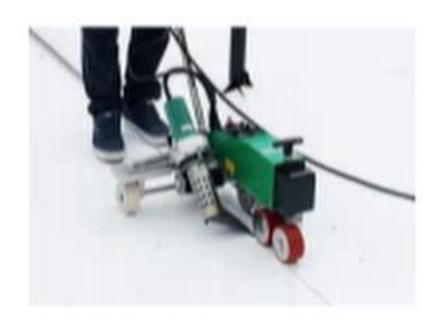
Easy to handle and user friendly due to optimal design and balance. Work now even more efficient with the LarOn 21, the fastest automatic welding machine in the market. You choose your optimum welding speed anywhere between 0,5–21 m/min.
